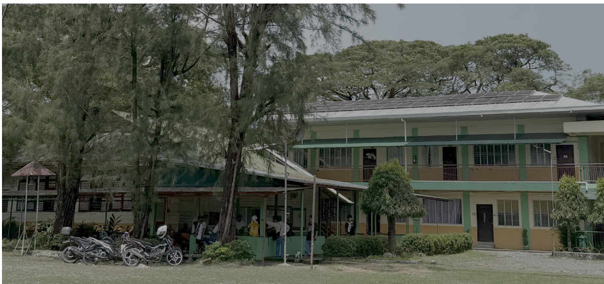
Solar power systems installed in Sacred Heart Academy in Gloria, Oriental Mindoro (top) and Holy Family Academy in Central, San Jose, Occidental Mindoro (bottom).
